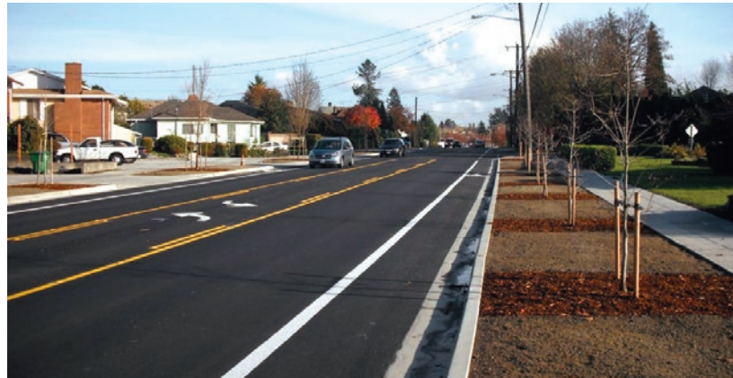
The project on this street in Seattle, WA added a new curb, street trees and a buffer between traffic and pedestrians. Photos courtesy of the National Complete Streets Coalition.
