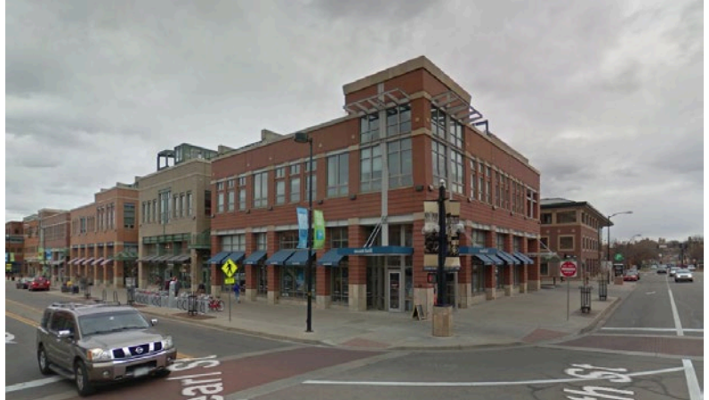
Parking structure at 15th & Pearl in Boulder, CO is wrapped by retail, creating a more vibrant pedestrian area. Imagery via Google Maps.
